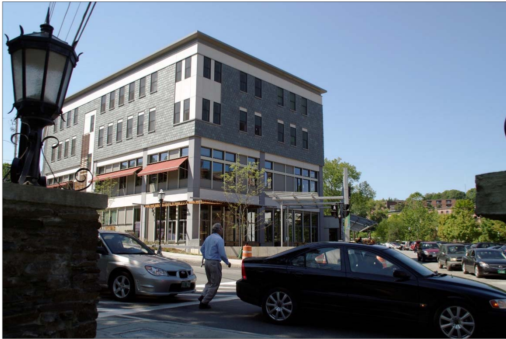
Canal and Main Apartments, Brattleboro 24 new construction apartments above the Brattleboro Food Co-op
