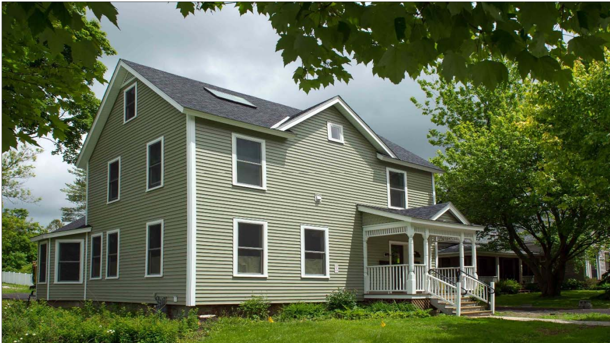
Rail City Apartments, St. Albans Scattered site renovations of 31 apartments
